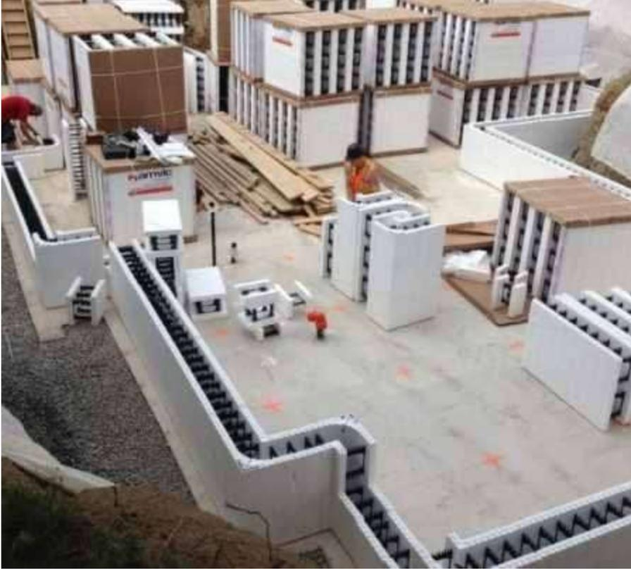
Fig 5: Insulated Concrete Forms
