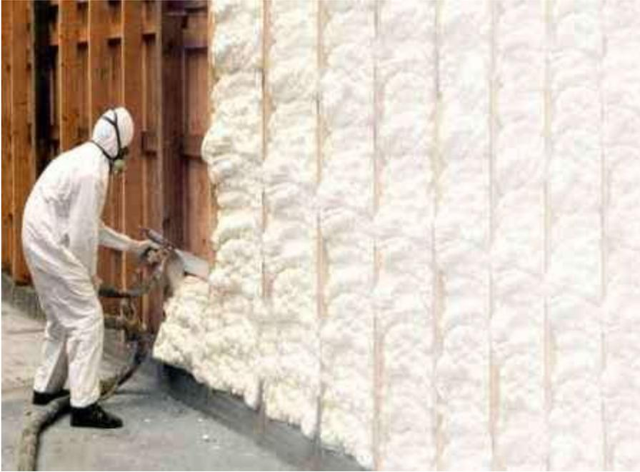
Fig 14: Polyurethane Foam Spray
