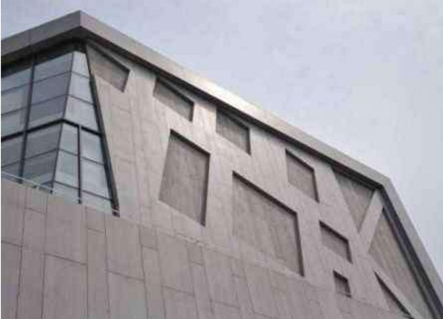
Fig 22: Exterior Siding with Fiber Cement Boards
