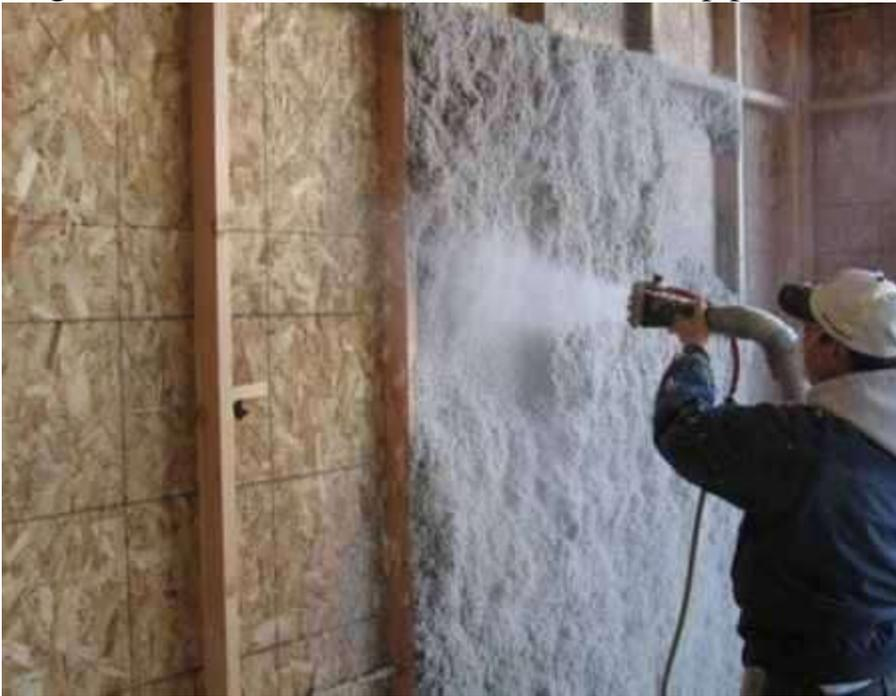
Fig 16: Installing Cellulose Insulation
