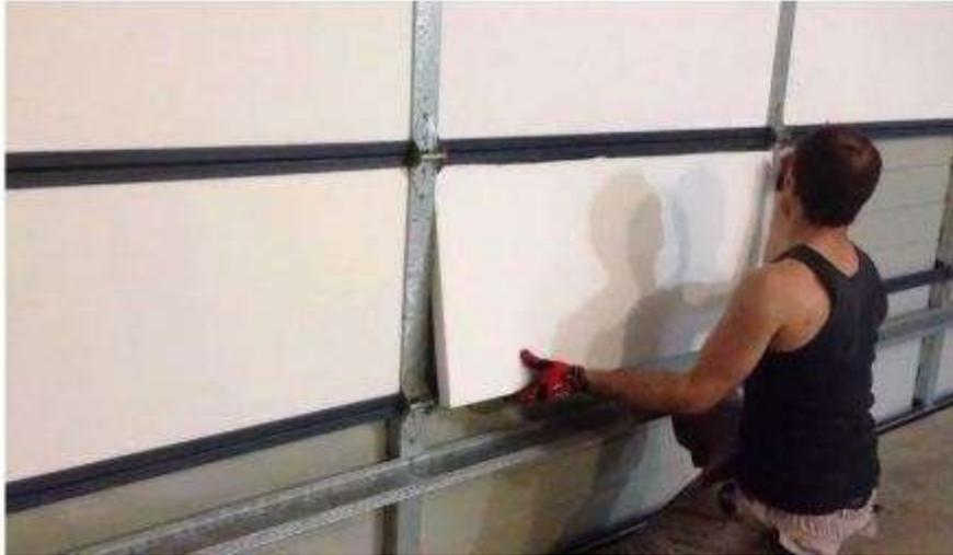
Fig 18: Installation of Polystyrene Foam Sheets
