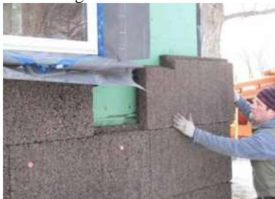
Fig 17: Installing Cork Boards
