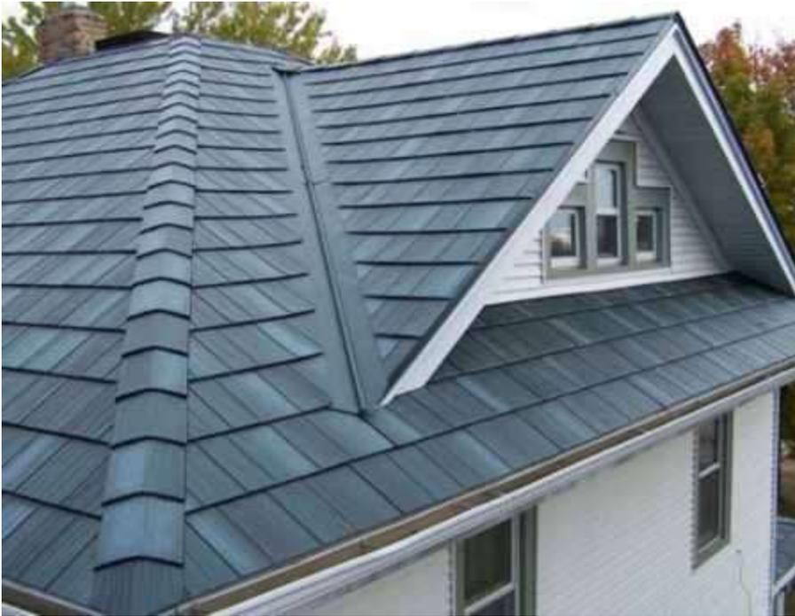
Fig 10: Steel Roofing
