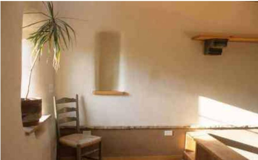
Fig 19: Natural Clay Plastered Wall
