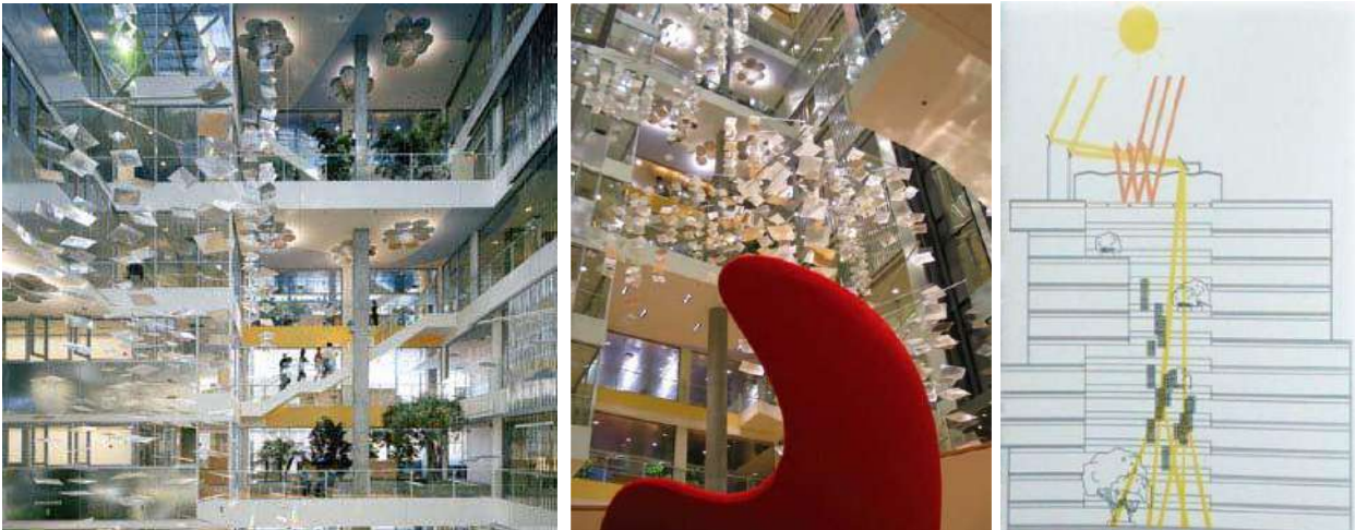
FIG. 2.12 Prisms being used to divert natural light inside the building.
