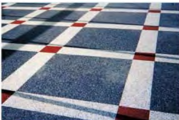
Red and blue pigments were used to color this terrazzo floor.
