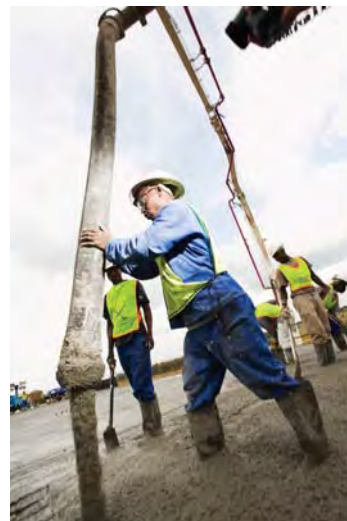
Self- compacting or consolidating concrete has many advantages
