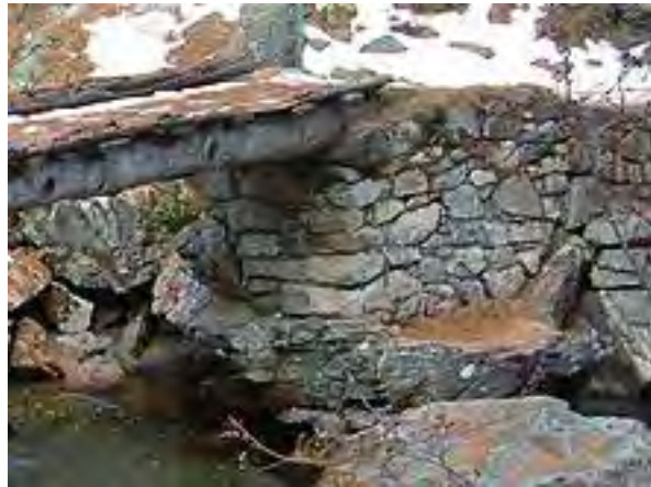
Dry set masonry supports a rustic log bridge, where it provides a well-drained support for the log (which will increase its service life)
