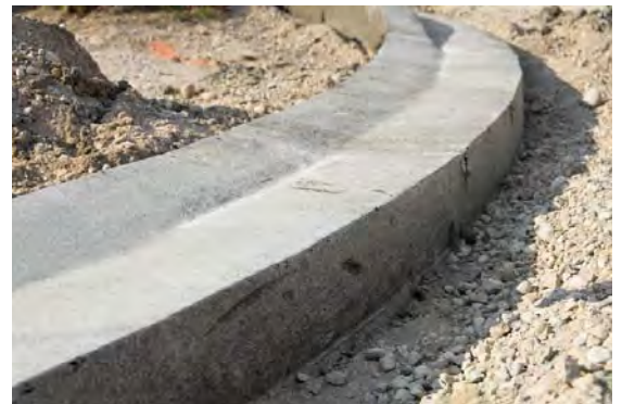
Uses, Benefits and drawbacks of fly ash in construction
