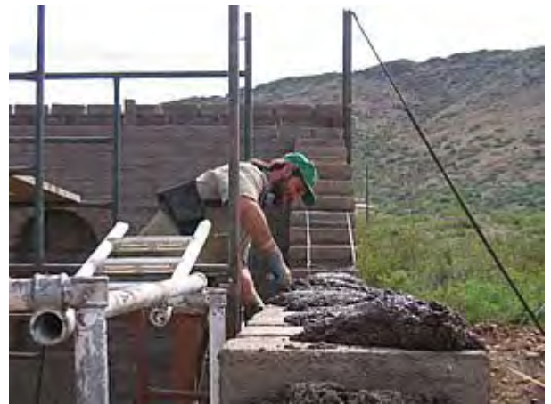
A mason laying mortar on top of a finished course of blocks, prior to placing the next course
