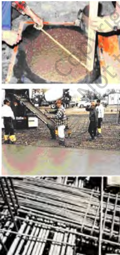
Flowable concrete with a high slump (top) is easily placed (middle) even in areas of heavy reinforcing steel congestion (bottom)
